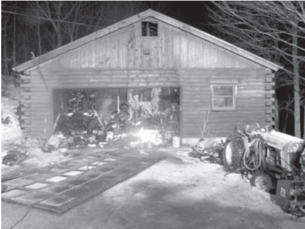
A Christmas night fire ravaged a garage at a house on Shoddy Mill Road, heavily damaging a motorcycle and Corvette.
