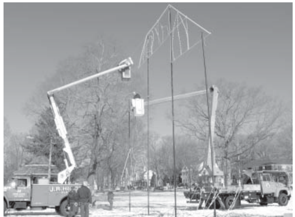
Personnel in two bucket trucks assembled a 39-foot rose on the town green Monday to promote the upcoming Colchester Community Theater production of Disney's Beauty and the Beast .
