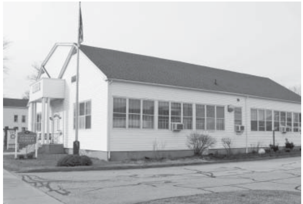
The Senior Center Study Group was recently extended for another year. The group is expected to make its recommendation for the future of Colchester’s senior center, pictured above, in about six months.
