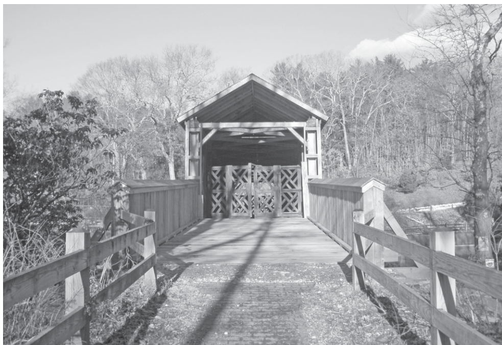
The Comstock Bridge, which spans the Salmon River from East Hampton to Colchester, is expected to completely reopen next month after a two-year renovation project. The bridge was built in 1873 and is one of only three remaining covered bridges in Connecticut.
