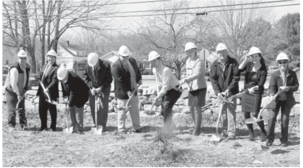
On April 4, a groundbreaking ceremony celebrated the start of construction of a new CVS/pharmacy in Hebron. Pictured here taking the first dig are, from left, town wetlands enforcement officer John Soderberg, property owner William Fochi Jr., Town Planner Mike O’Leary, Roger Adams with the Windham Regional Chamber of Commerce, Town Manager Andy Tierney, CVS/Caremark district manager Tim Roy, state Sen. Cathy Osten, property owner William Fochi Sr., CVS/Caremark district supervisor Jennifer Nemeec and selectwoman Gayle Mulligan.
