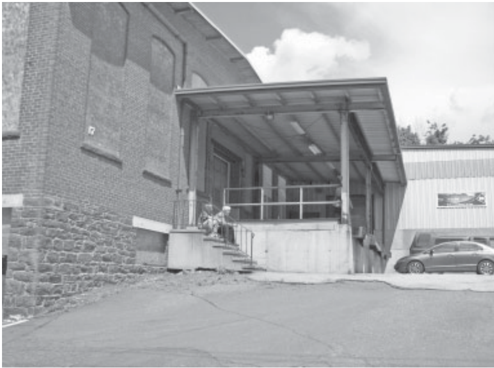
After being destroyed by a fire about one year ago, the Bevin Bell factory was forced to relocate. Pictured above is the building on Watrous Street, out of which the company is operating indefinitely.
