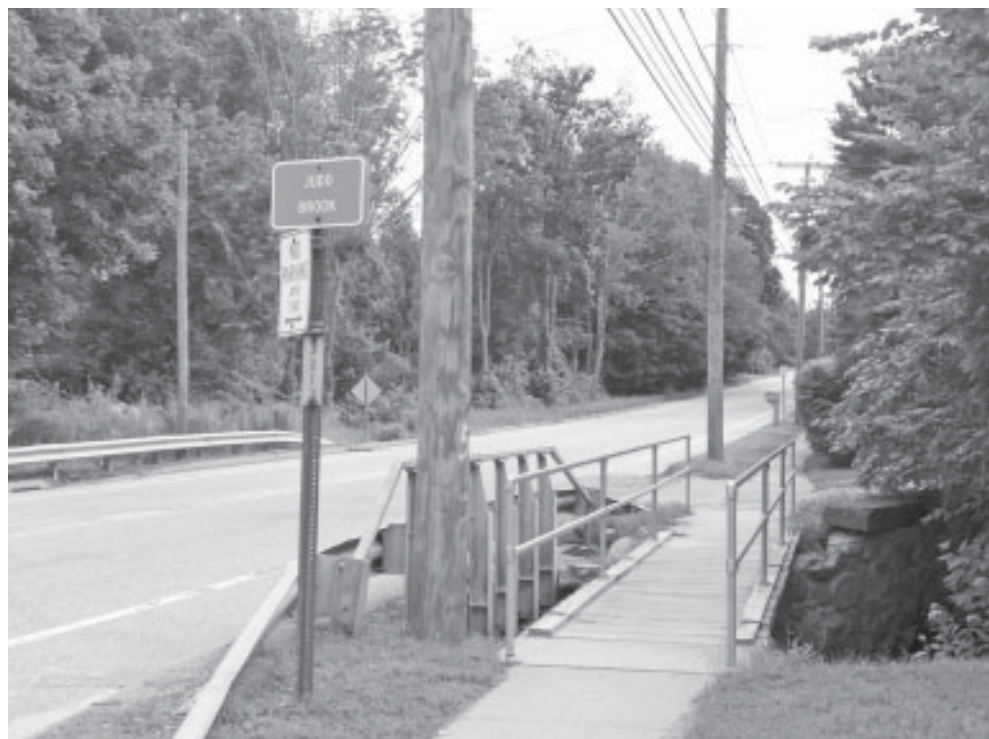
Judd Brook – shown here running under a Norwich Avenue bridge – plays a key role in a lawsuit filed against the town by residents Victor and Olga Wozniak. The couple is suing Colchester for failing to correct its Flood Insurance Rate Map (FIRM) that incorrectly places the brook on a portion of their property on Lebanon Avenue.
