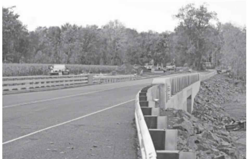
**The Carr Brook Bridge on Route 17A reopened Tuesday afternoon after five months of construction work. Renovations replaced the bridge entirely with a newer design, expanded the bridge and road width, added new guardrails and resurfaced 500 feet of road on and around the bridge.**
