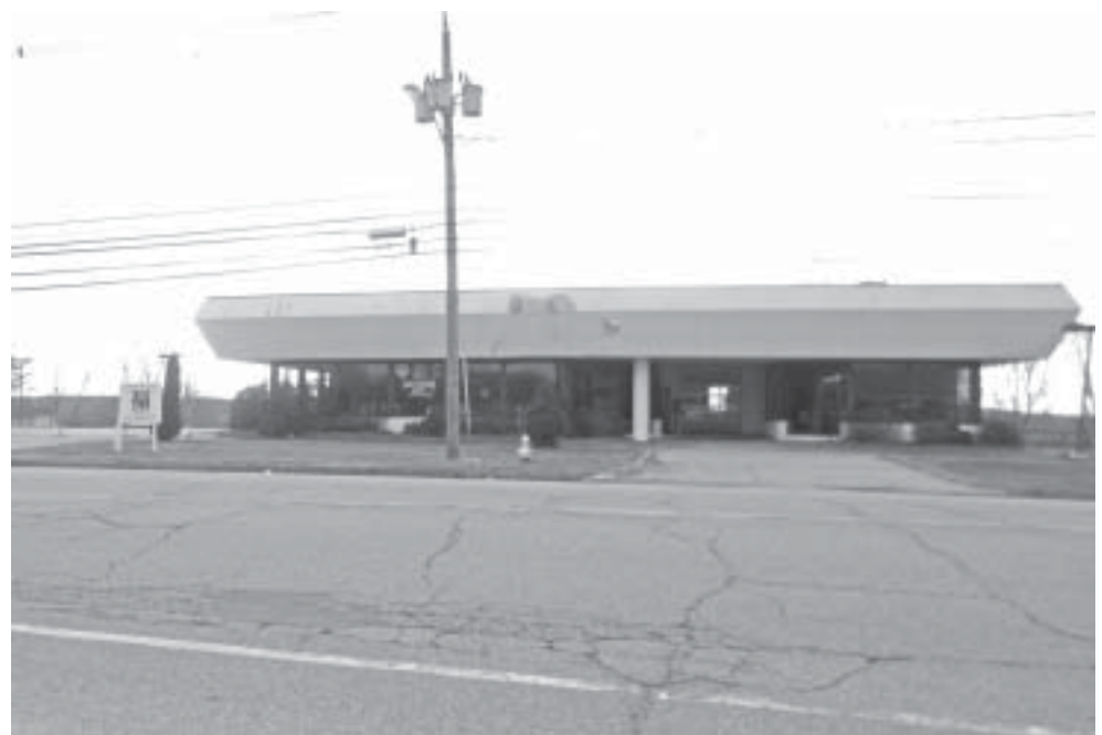
The former Jack's Chevrolet property at 120 South Main St. has been vacant since the dealership's closing in June 2009. It may soon be sold – and replaced by a pharmacy and restaurant.
