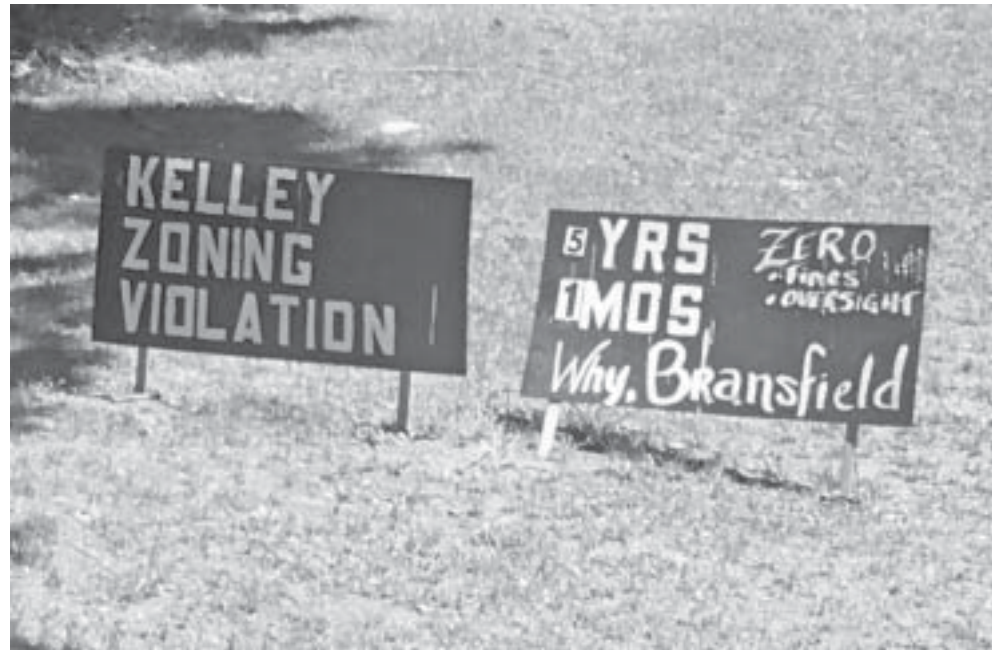
Melissa Gerrier-Satagaj and Bob Satagaj placed signs in their yard to protest their neighbors' paved driveway, which has been causing flooding and erosion issues for five years despite a former zoning enforcement officer's 2013 order for the owners to replace it with gravel.
