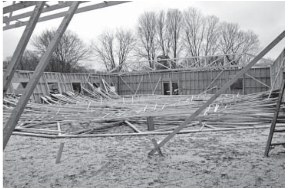
A crane was lifting large trusses onto the 12-foot-high walls of the building when the trusses fell into the structure, officials said. Investigations by local, state and federal agencies are working to determine what caused the collapse and whether or not the remaining walls are structurally sound. Photo credit: East Hampton Building Department
