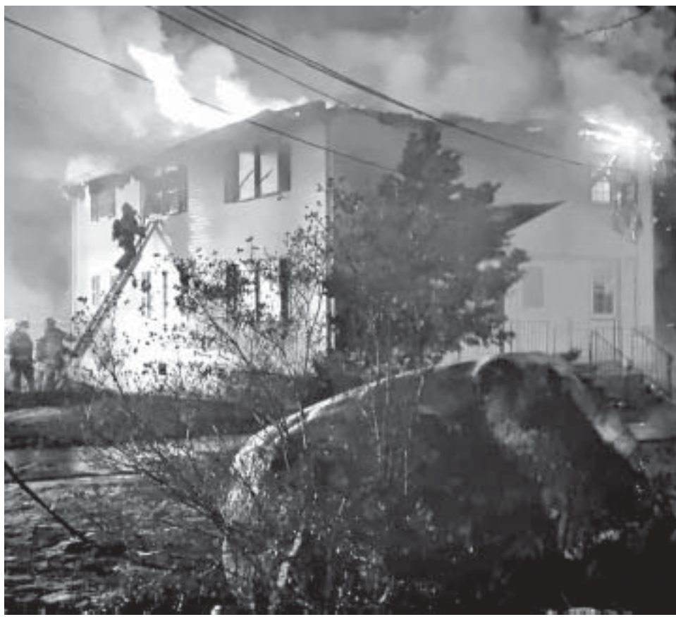
Fire Ravages Home... An East Hampton duplex was ravaged by fire Sunday night. Everyone was able to safely escape the blaze, and no injuries were reported. See story on page 19.
