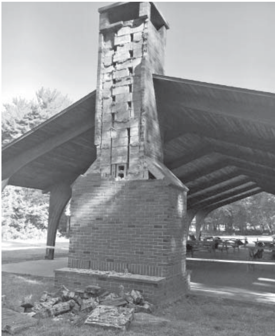
Fire Causes Explosion... A homemade fire in the chimney at the Blish Park pavilion in Marlborough July 24 led to a small explosion. According to police, five teens gathered sticks to make a fire, and everything appeared normal until an explosion occurred inside the chimney, causing chunks of brick to fly off. The future of the chimney, including potential repairs, was discussed at this week's Board of Selectmen meeting. Photo courtesy of Amy Traversa. See story on page 9.
