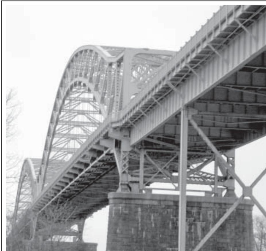
**Bridge Work to Start...** Motorists will be affected when a construction project on the Arrigoni Bridge starts Feb. 27. Work will include replacing bridge decks, superstructure steel upgrades and repairs as well as substructure repairs designed to improve overall structural capacity, reliability and integrity of the bridge. For more on the project, see a story on page 12.
