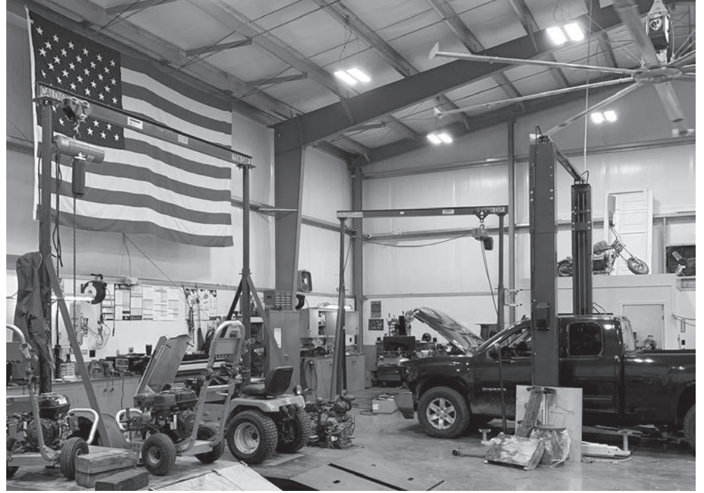
The new service shop at Gano's is all-American – in every sense of the word. Each part of the new shop – from the lights down to the radiant floor heater – is all made in the U.S.A.
