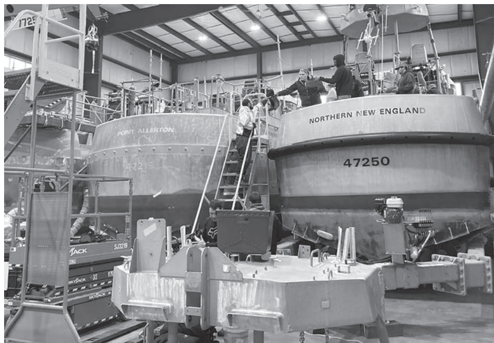
U.S. Coast Guard Station South Portland and Sector staff recently dropped off one of their 47-foot motor lifeboats (MLB) at the new Birdon facility on the Connecticut River in Portland.
