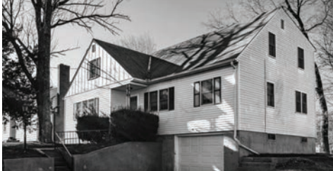
61 Ridge Rd, Middletown Tyler DeVecchis 860-966-9217
