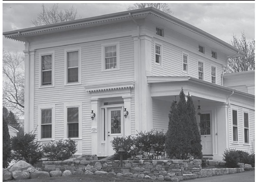
One of the six homes on the CHS Historic House Tour is the c. 1855 Strong-Chapman House on South Main Street. A tavern once sat on this property run by David Strong. This cube shaped home with Italianate style eaves and elaborate cornices has been renovated. Photo by Maggy Morales.
