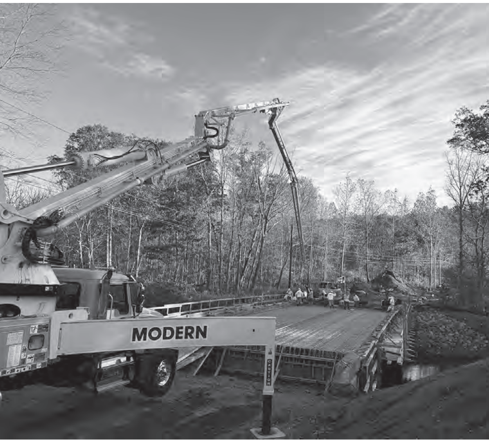
Modern Concrete Pumping, Inc., owned by Andover resident Marcus King, is helping complete work on the new Bunker Hill Bridge. Once the project wraps up, the road will officially reopen – allowing school buses and local traffic to travel safely down Bunker Hill Road for the first time in a very long time.
